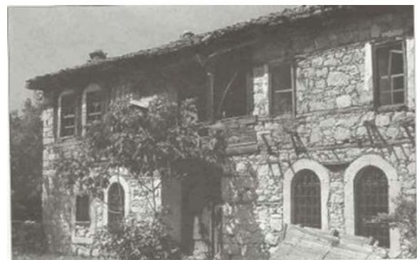
Fig. 6: Bigadiç's single manner of construction
