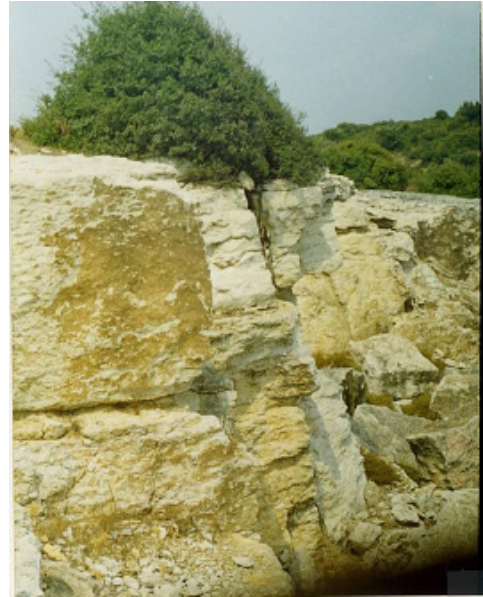
Fig. 2. Thick layered limestones in the east of Yeniçiftlik and their disintegration into smaller blocks starting from the surface.
