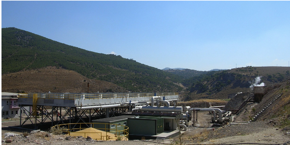
Fig. 2. Tuzla geothermal power plant.
