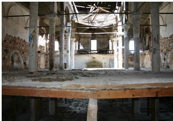
Figure 5. Inside Hagia Triada Church (İnce Güney, 2007)
