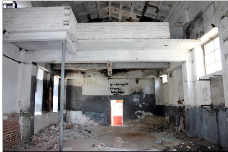
Figure 4. Inside of Feneromeni Church (İnce Güney, 2007)
