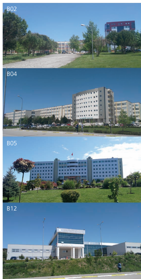
Figure 3. Views of the Faculty of Engineering and Architecture (B02), Faculty of Arts and Sciences (B04), rectorate building (B05) and School of Physical Education and Sports (B12)
