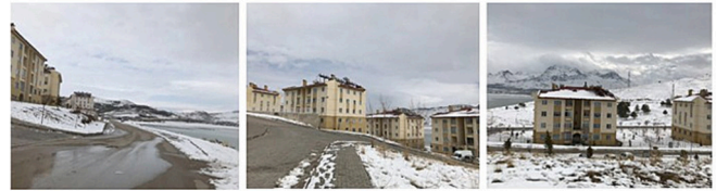
Figure 2b. Akköprü Permanent Housing Settlement
