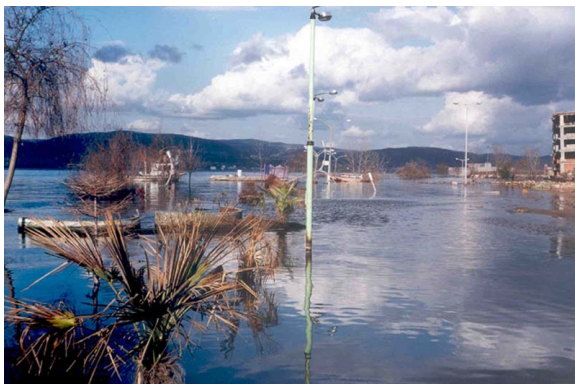
Fig.2. Inundation by seawater due to coastal subsidence near Gölcük
