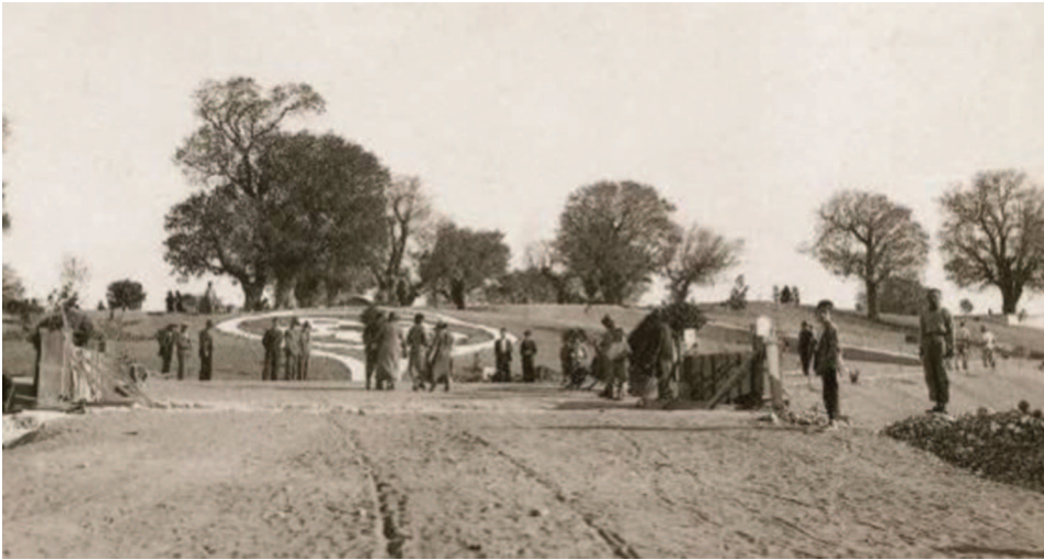
Figure 5. ‘Atatürk Medallion’ and Ceremonial Square under construction (Faruk Ergelen Archive).
